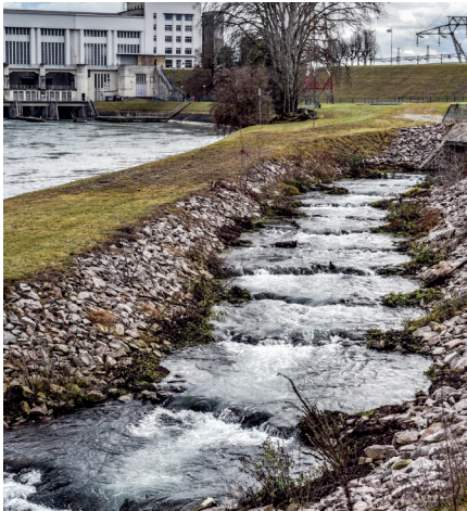
A fish ladder ensures that fish securely bypass a dam on the Rhine.
